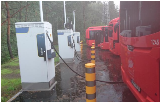
Klemetsrud 50 kW plugg
