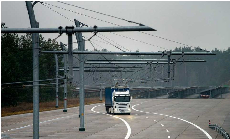
Figur 3.3: Infrastruktur for Siemens eHighway. Foto: InsideEVs.com
